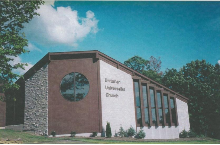
Fee Lane meeting hall (sanctuary) addition and offices (1998-present) seen from the north
