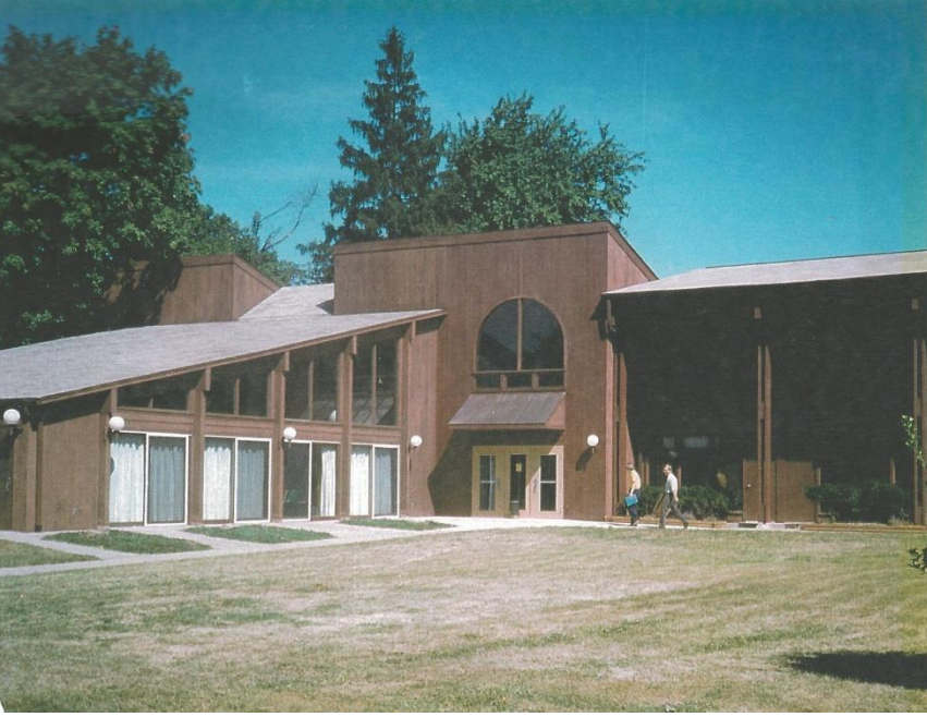
Figure 6-1 The Fee Lane addition and remodeling (1975-1998)
