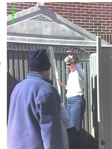
Angela Lexmond helps build storage shed
