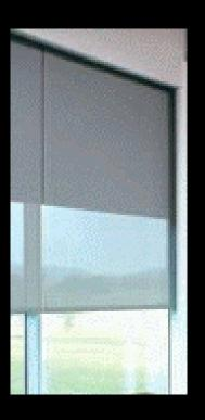
A second shade, installed in the same fascia box, could be lowered to block light for projections during service or during music or theater events. They could be separately controlled.
