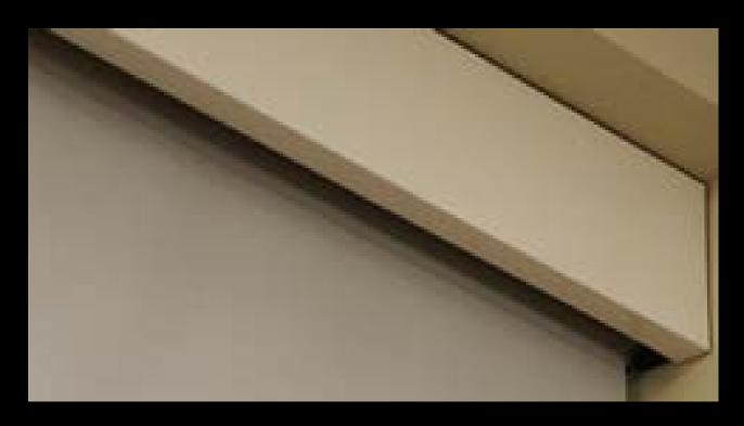
A small fascia box, painted to match the wood, would be mounted at the top of the wall above the round window, so the shade would be out of sight when not deployed.
